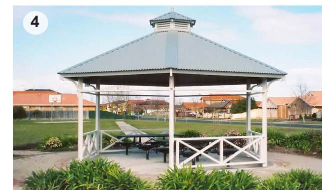
4 CIRCULAR PARKLAND SHELTER FACILITIES
